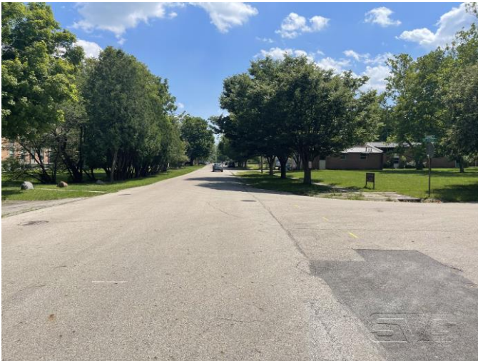
Street View South – Livermore St.
