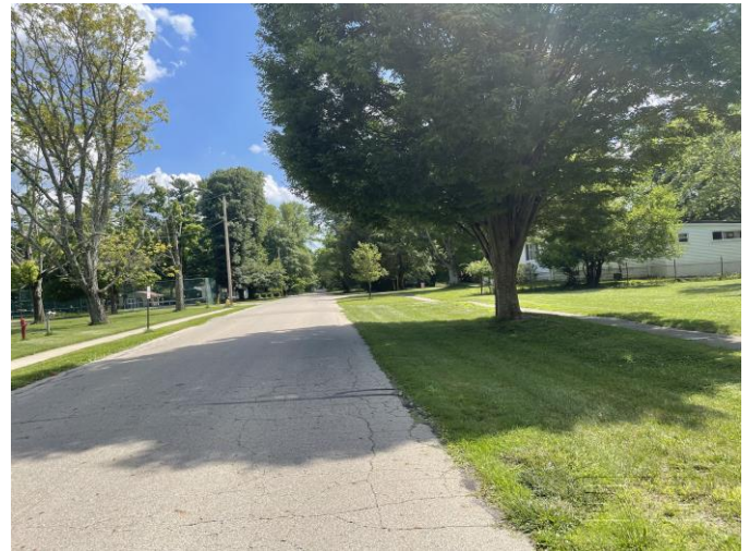
Street View - South- Livermore Street
