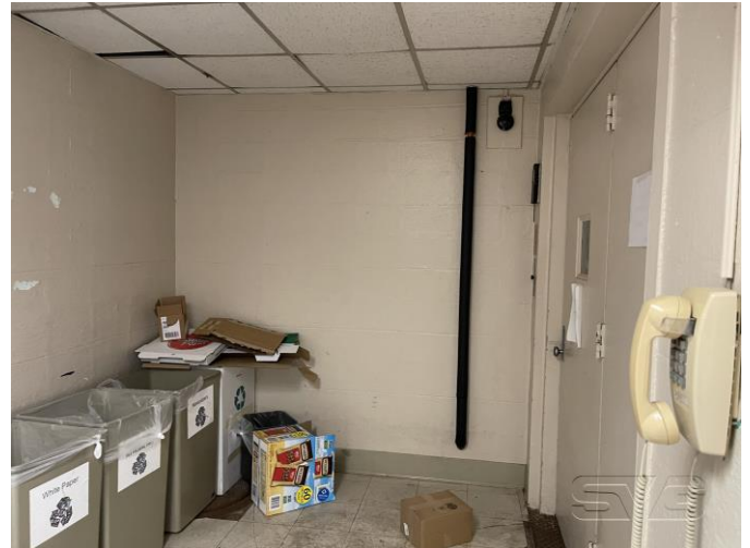
Interior– First Floor
