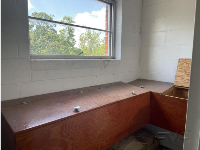
Interior– Roof Floor
