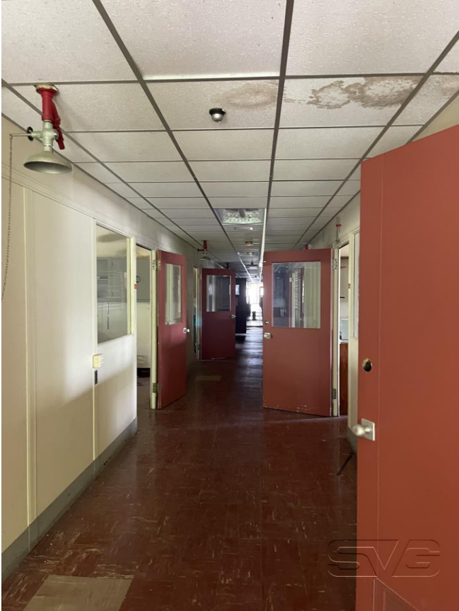
Interior– Third Floor
