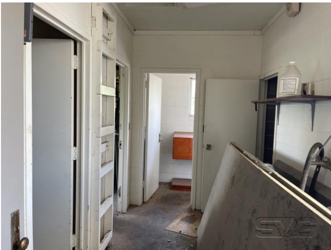
Interior– Roof Floor
