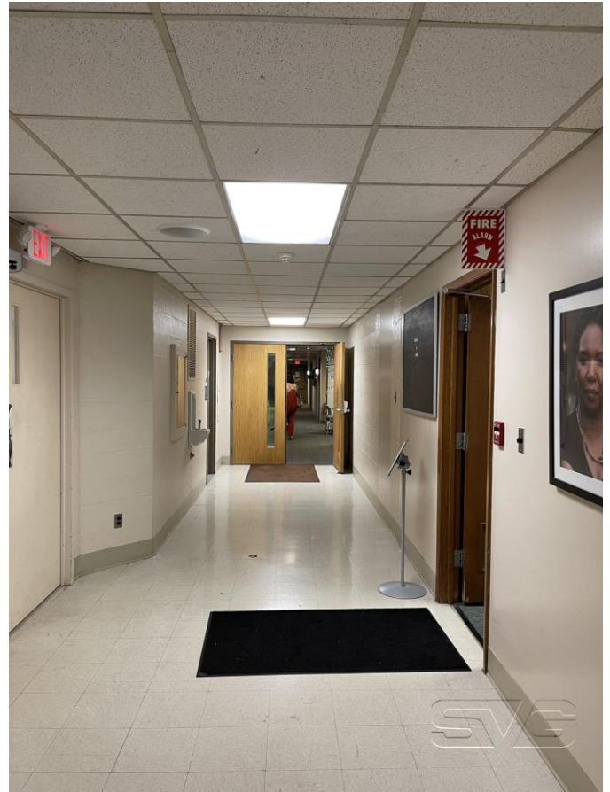
Interior– First Floor
