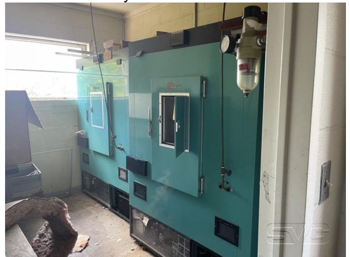
Interior– Roof Floor
