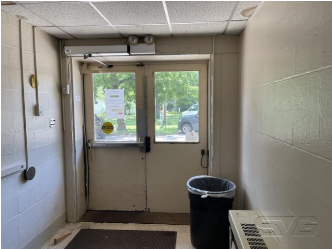
Interior– First Floor
