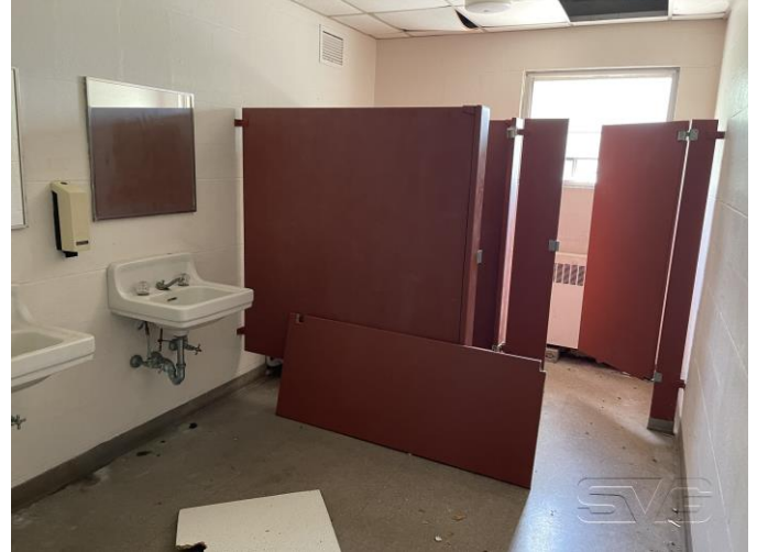
Interior– Third Floor
