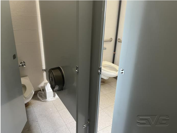
Interior– First Floor
