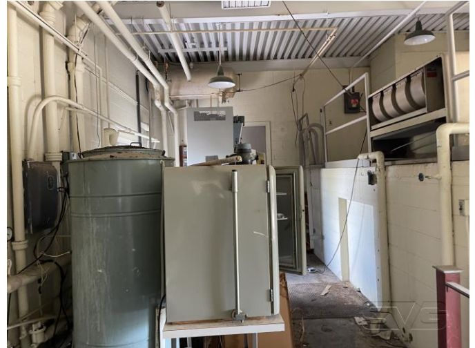
Interior– Roof Floor
