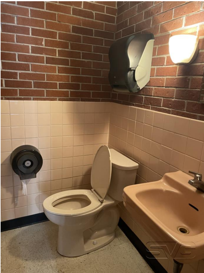
Physical Plant – Interior – Bathroom
