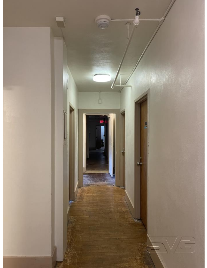
Interior – Second Floor - Hallway
