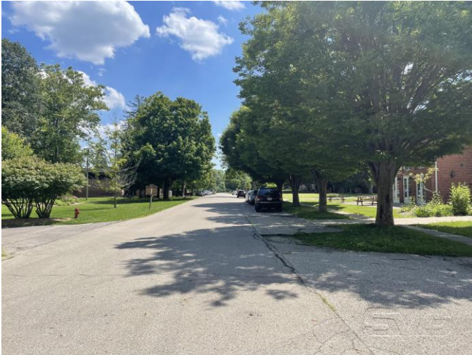
Street View – Livermore Street - South
