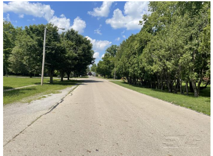
Street View – Livermore Street - North
