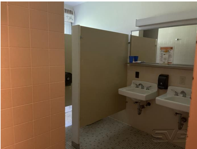
Interior – Second Floor - Bathroom
