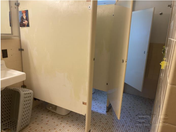
Interior – Second Floor -Bathroom
