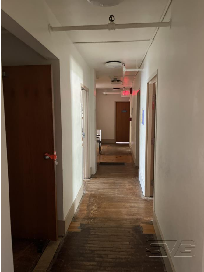
Interior – First Floor – Hallway
