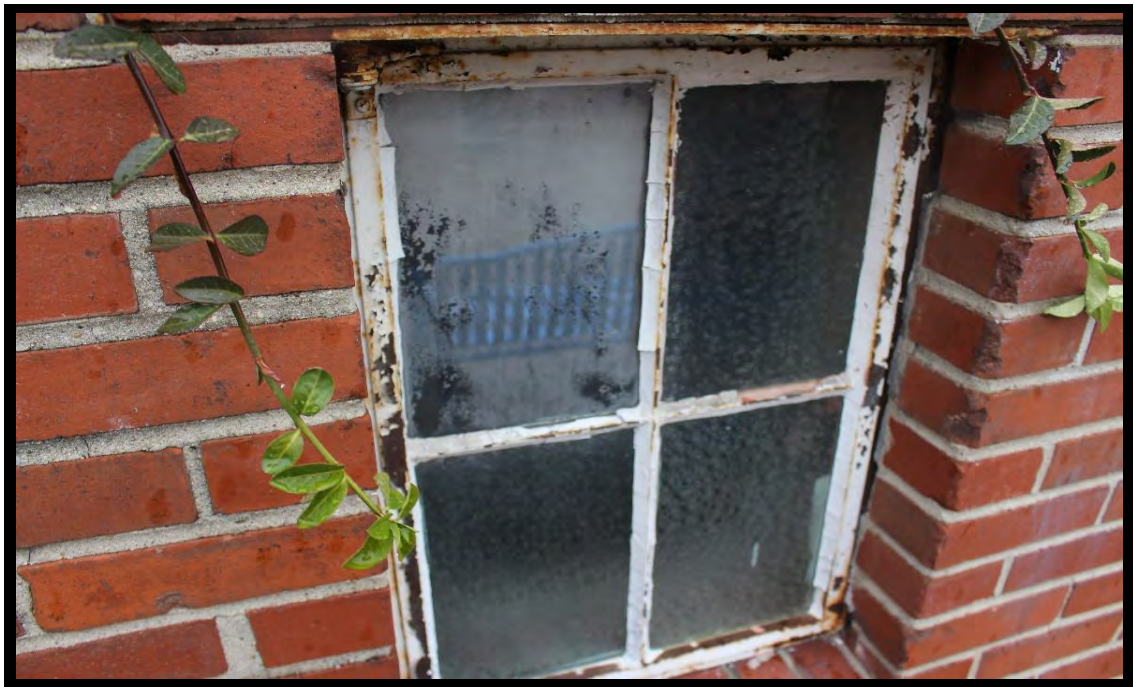
6 All the windows in both buildings appear to be original. Metal windows on the first floor, and wooden windows on the 2nd and 3rd floors. All windows have window glazing in poor condition.
