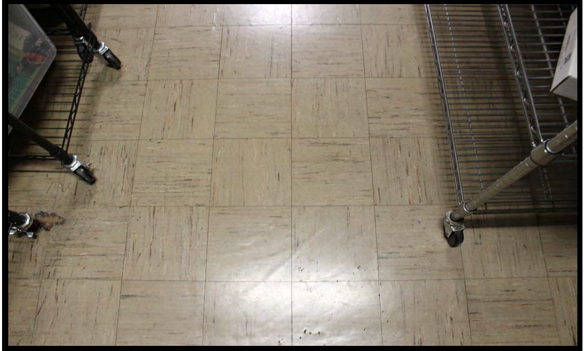
15 A storage room with 9x9 vinyl floor tiles.
