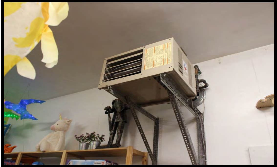
13 The overhead gas space heater in the toy store.
